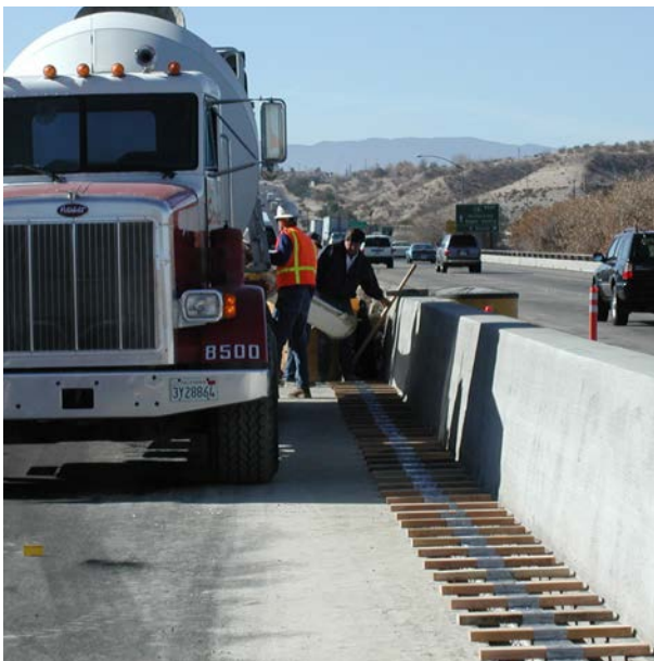
Highway barrier drainage
