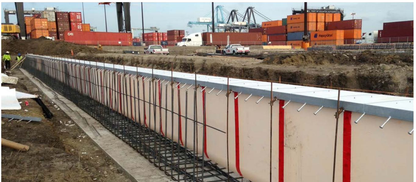
TrenchFormer XHD installed at the Port of Houston
